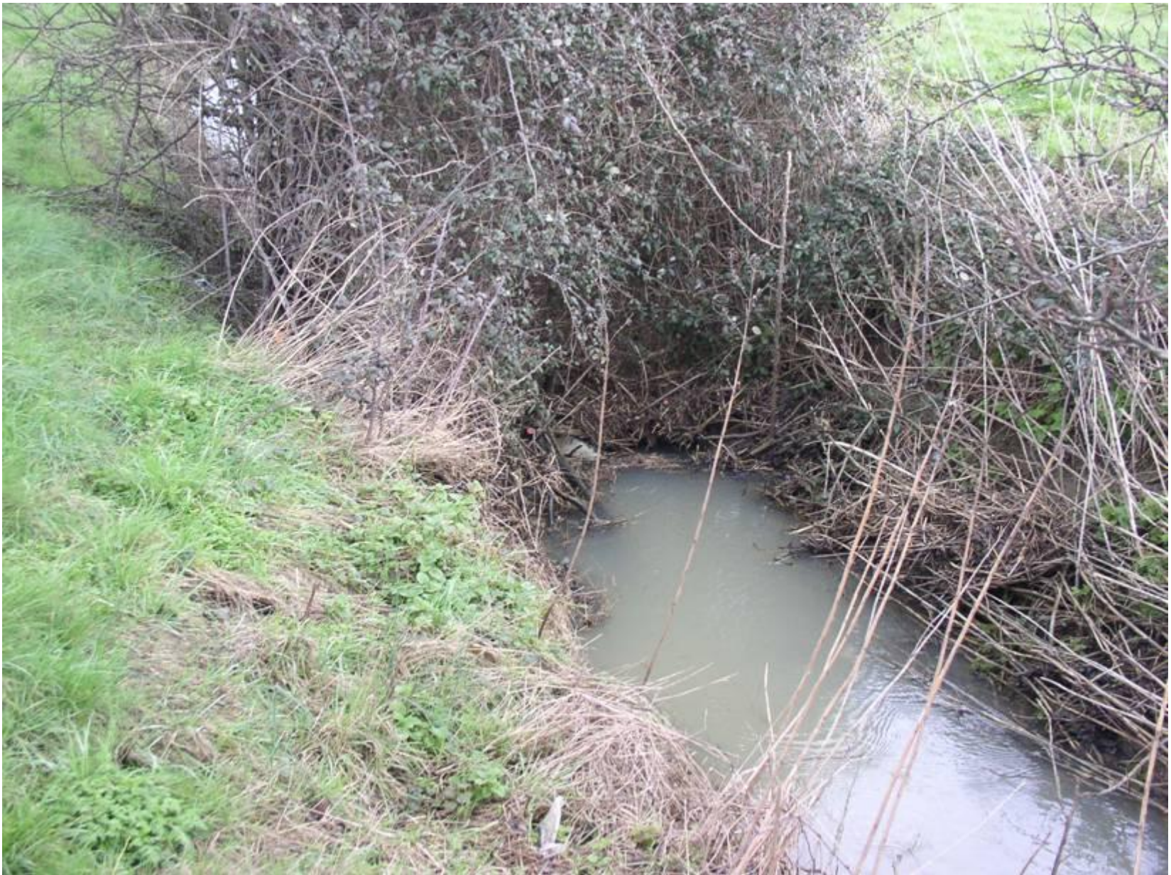
Build-up of natural debris + man-made items 150 metres north west of New Farm.
