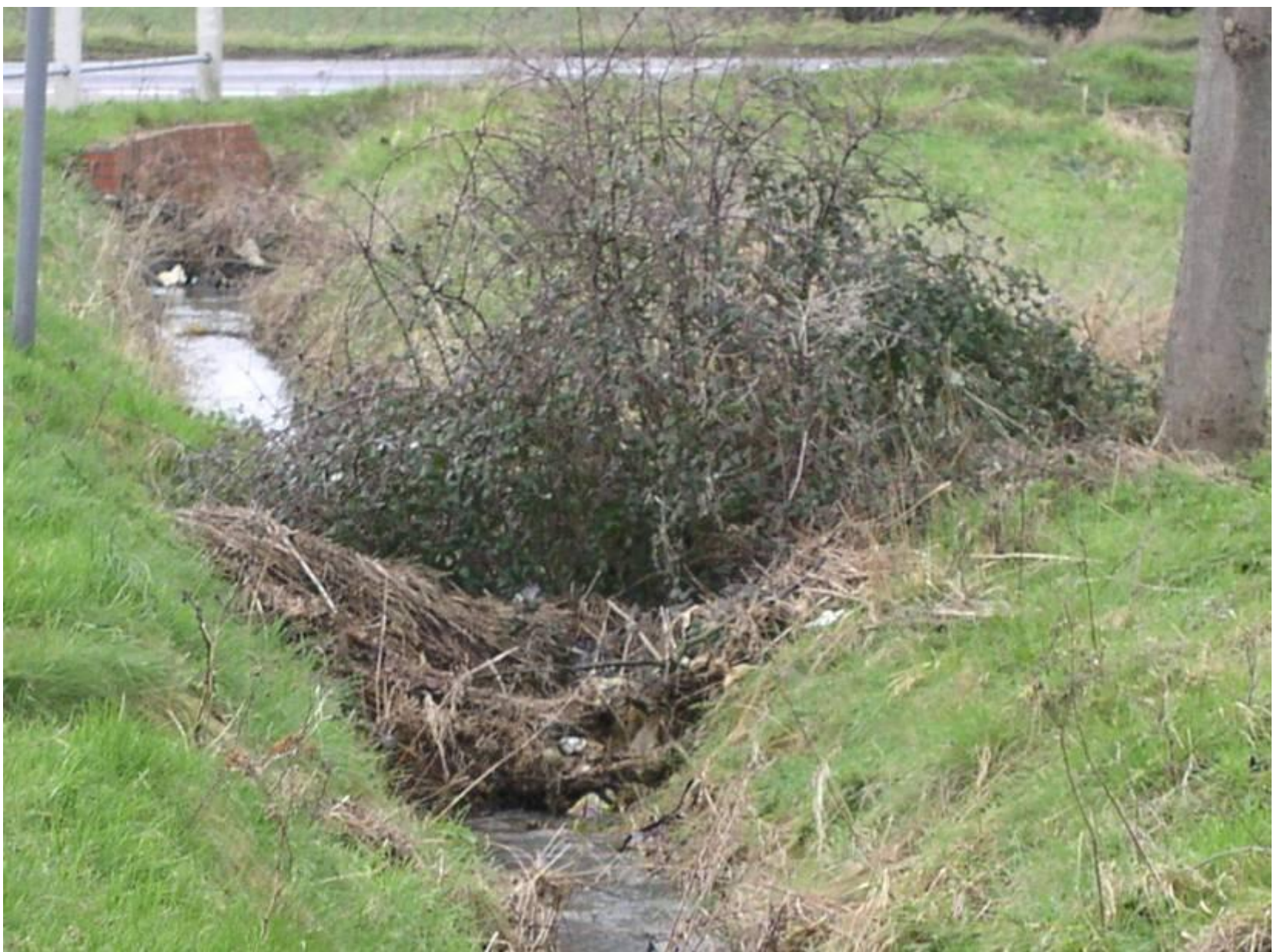
Area of natural debris build-up just east of B1040/Rogue's Lane junction. Although relatively severe, this was not causing any significant blockage.
