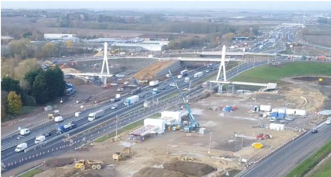
**Section 5:** The extensions to the bridges at Kings Hedges and Impington, pictured below, continue, with the installation of the beams to support the new carriageway and then laying the basecourse, water proofing across each bridge.
